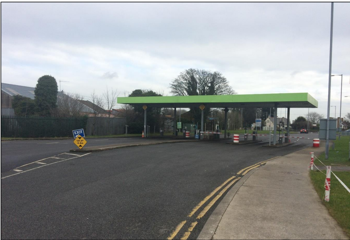
Fig 2 – Existing Canopy entrance and ticket barriers
